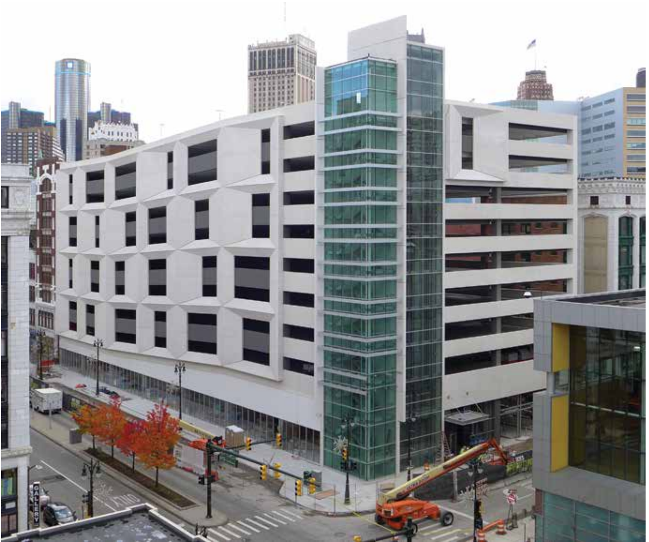
The Z, a 10-story, mixed-use property in Detroit includes a 1,282-car precast concrete parking structure designed with “picture-frame” style windows made with trapezoid-shaped spandrels and horizontal openings that band the structure. Additional lights and accents highlight the exterior; while murals enliven the interior. Photos: Neumann/Smith Architecture.
