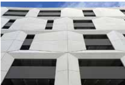
The Z, a 10-story, mixed-use property in Detroit includes a 1,282-car precast concrete parking structure designed with “picture-frame” style windows made with trapezoid-shaped spandrels and horizontal openings that band the structure. Additional lights and accents highlight the exterior; while murals enliven the interior. Photos: Neumann/Smith Architecture.
