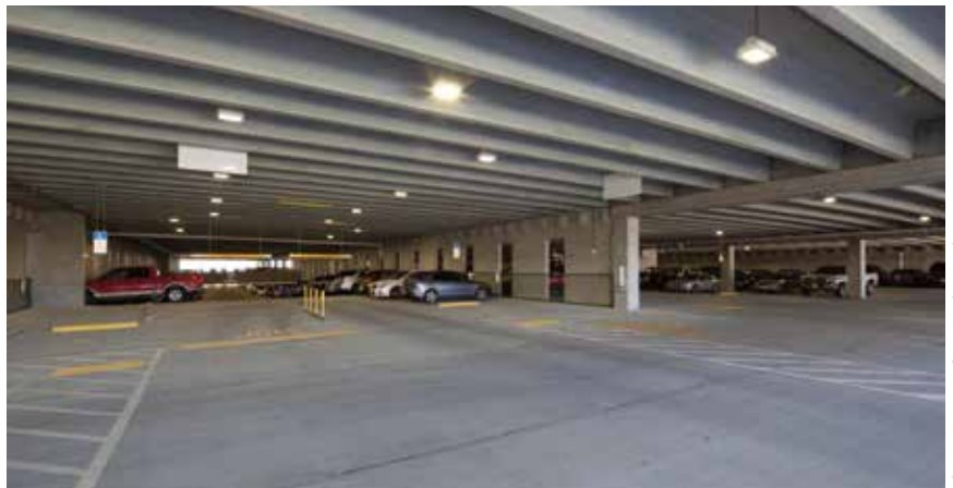
Photo: Lutz Prebor Fowler Architects.
