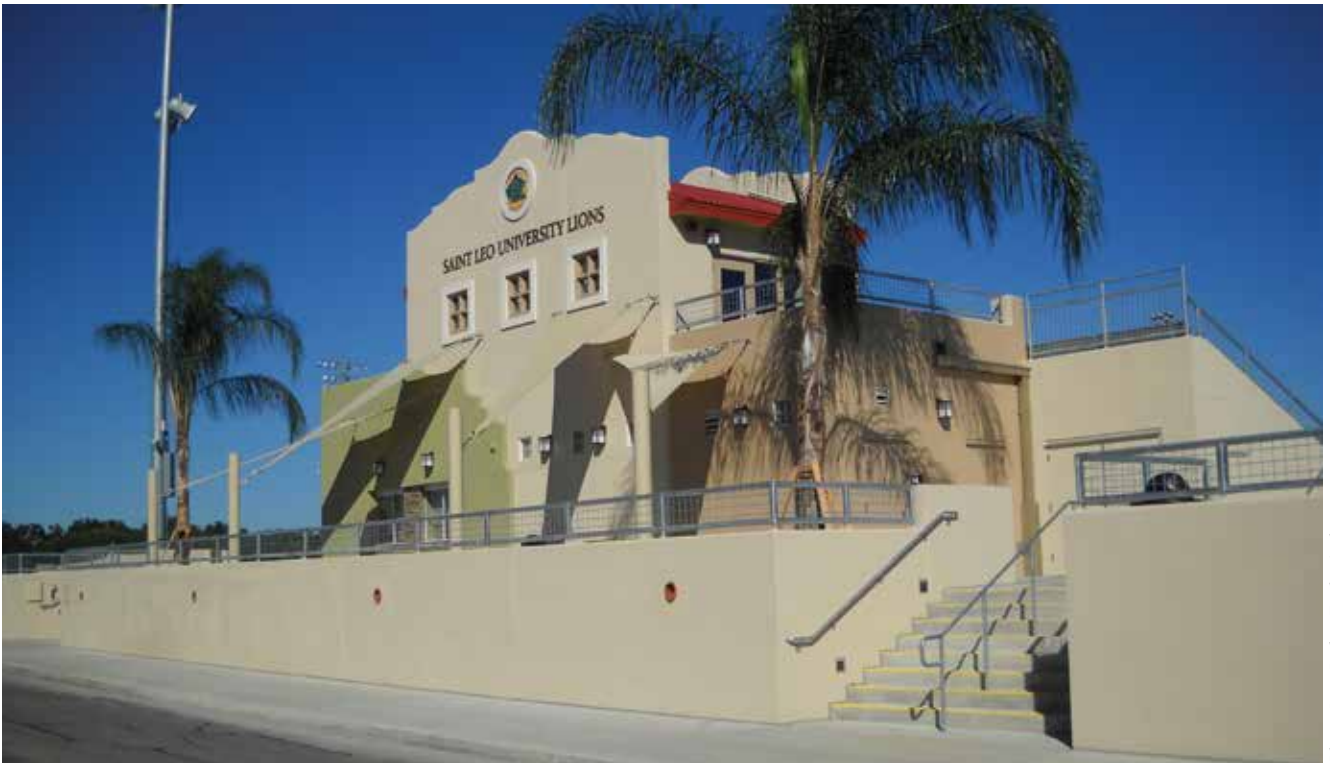
Photo: Lutz Prebor Fowler Architects.
