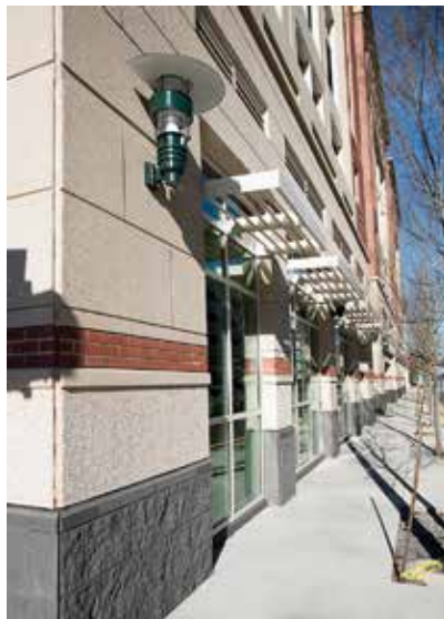
Cast stone block and thin brick were cast into the architectural precast concrete panels cladding the six-level, 524-car precast concrete parking structure at the City Center Development in Columbia, S.C. It helped transform a low-density surface parking lot in an urban, historic area into a high-density infill project. Photos: LS3P.
